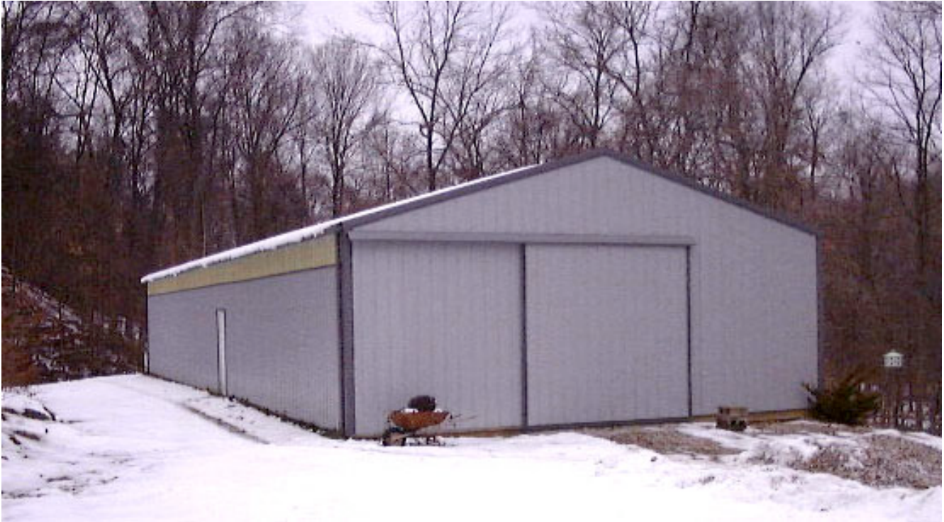
Amish Built Pole Barn
