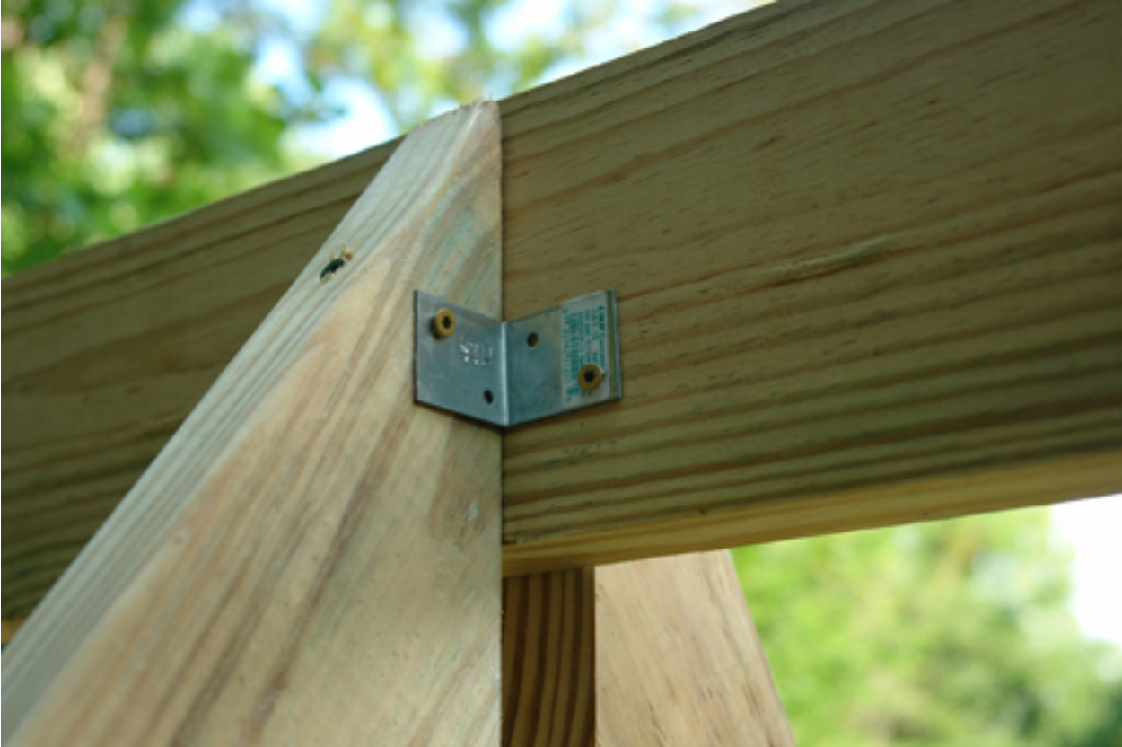
Joining roof rafter to roof ridge
