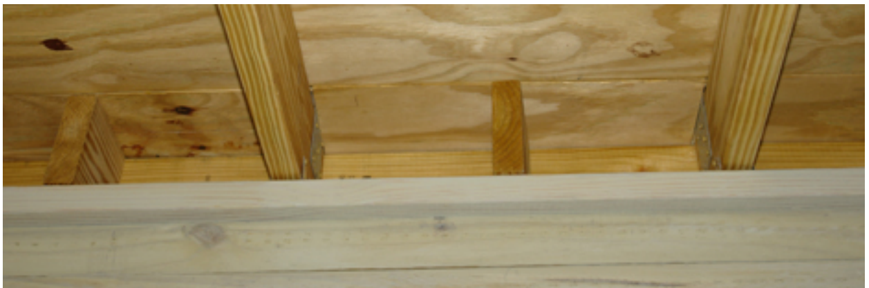
Plywood strips (bracing on underside)
