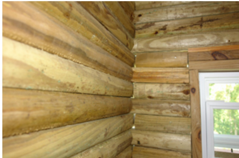
Air gap between logs
