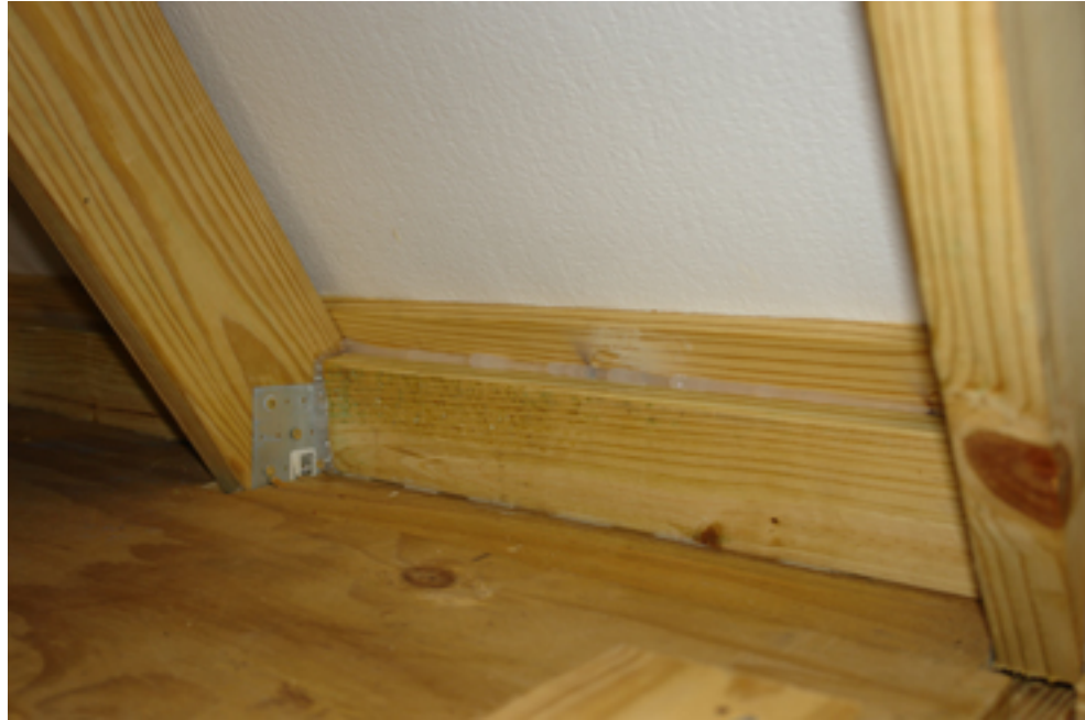
Plugging Air Gaps
