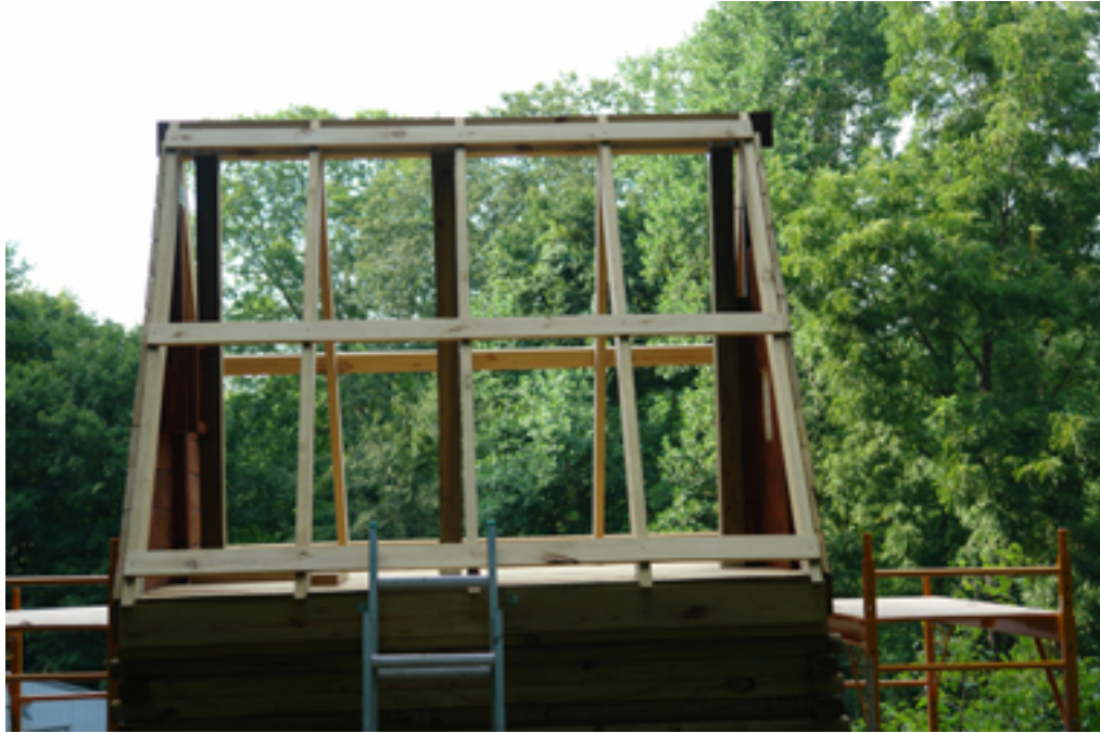
Wood Nailers (batten boards)
