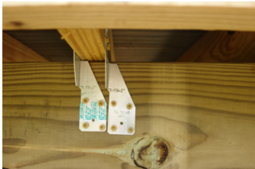
Attaching Joist to Beam
