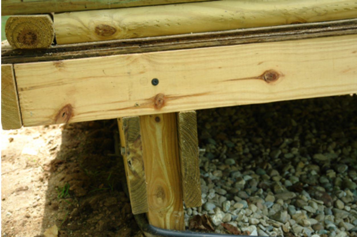
Attaching Beams and Floor Joist to Post
