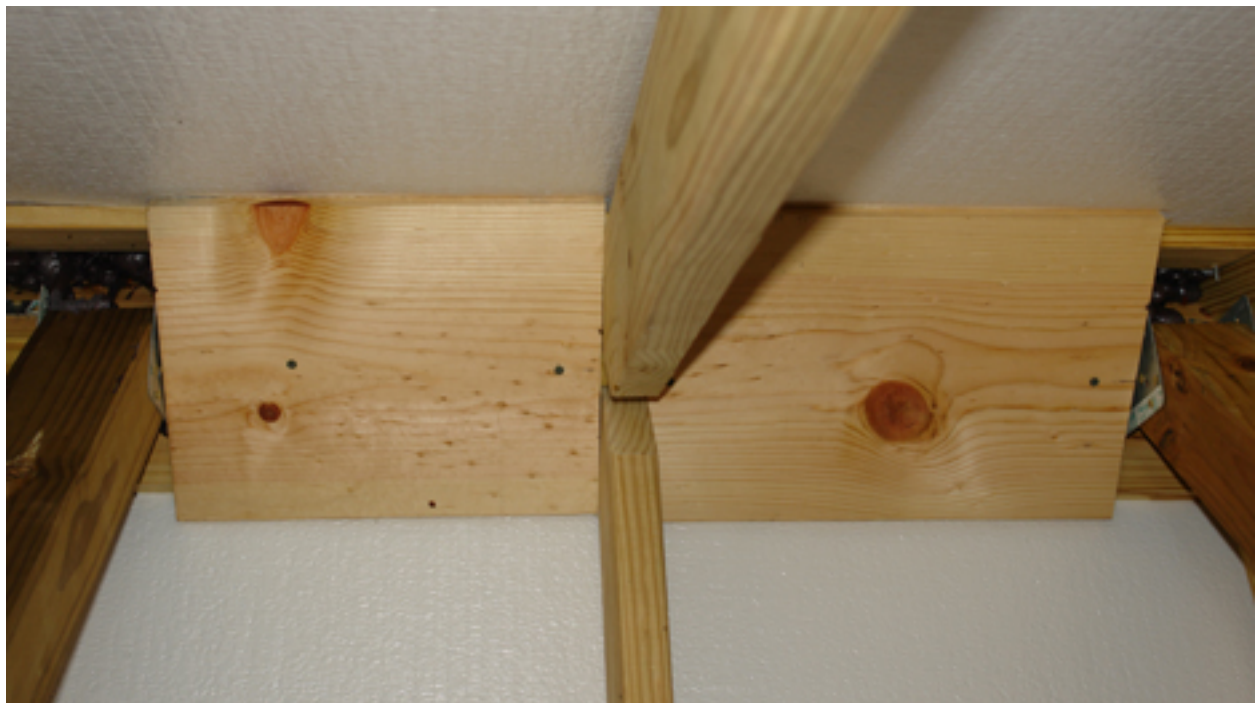
Sealing Roof Ridge
