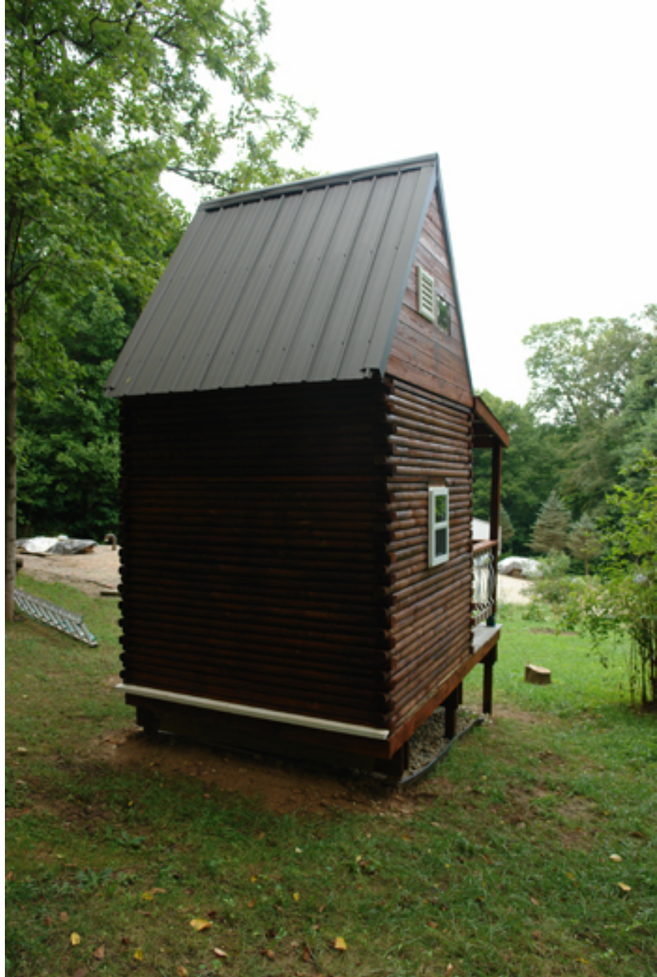
White PVC boards on plywood lip
