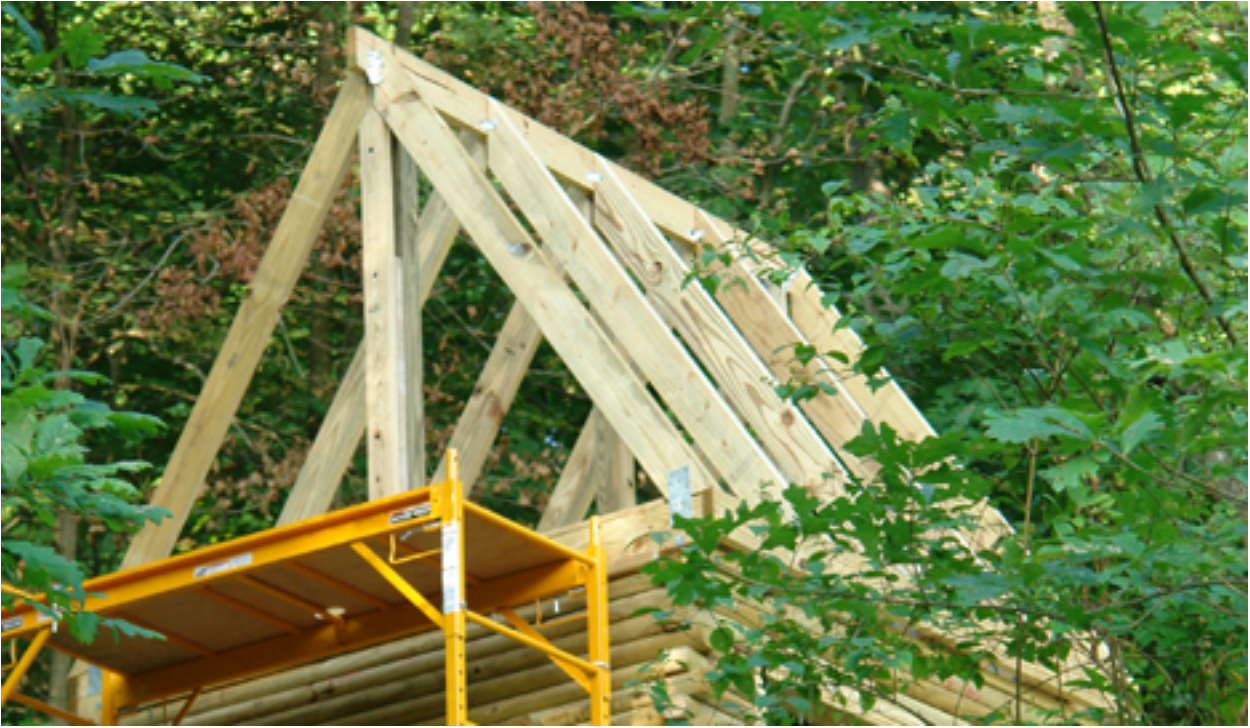
Installation of Roof Rafters
