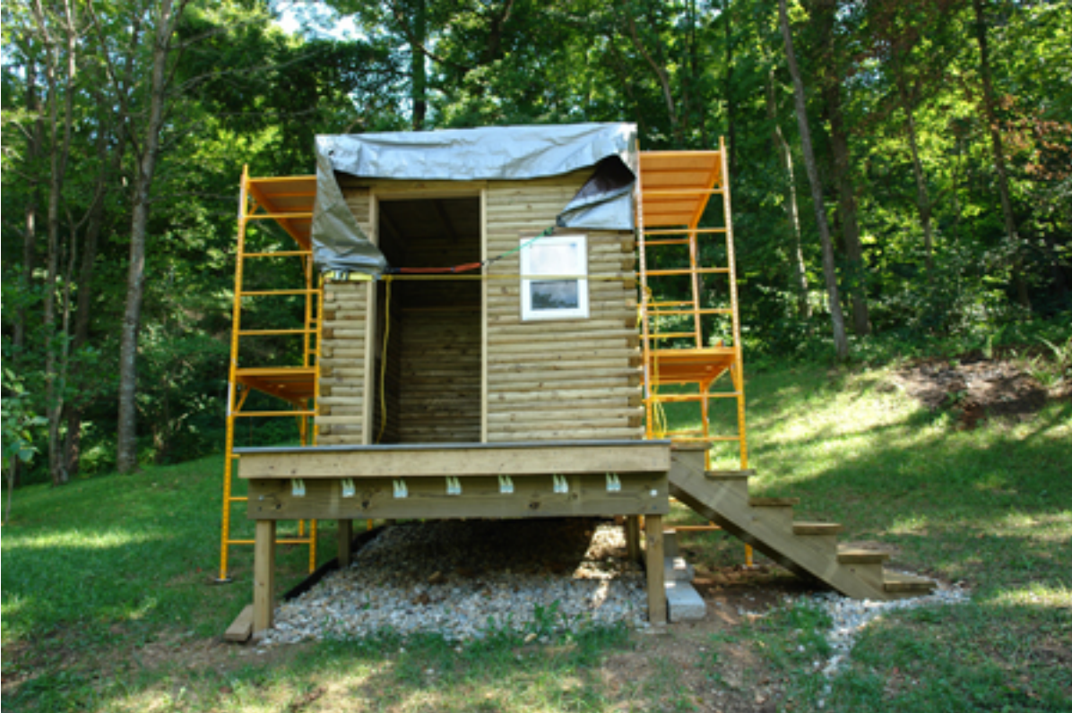
Anchoring Scaffolding
