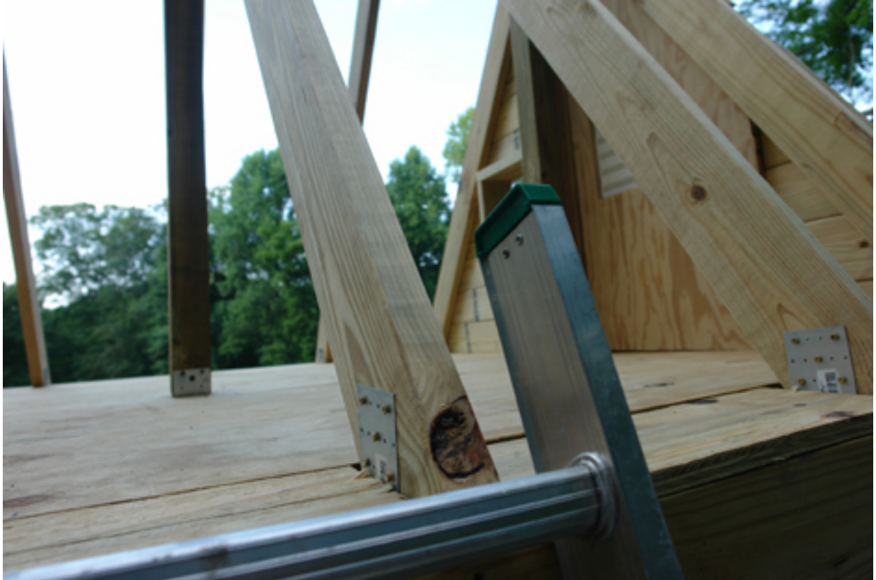
Plywood Strips (topside)
