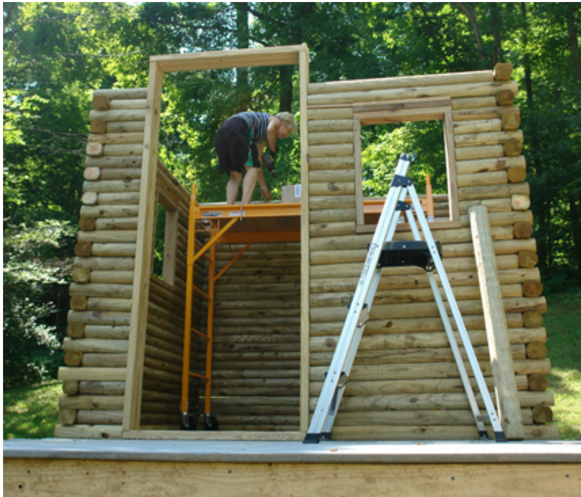
Leveling above window frame
