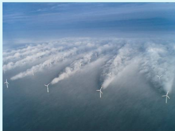
Illustration of wake effect at an offshore wind farm. Hasager et al. (2013), Energies , 6:696-716. Photo by Christian Steiness (via Vattenfall).
