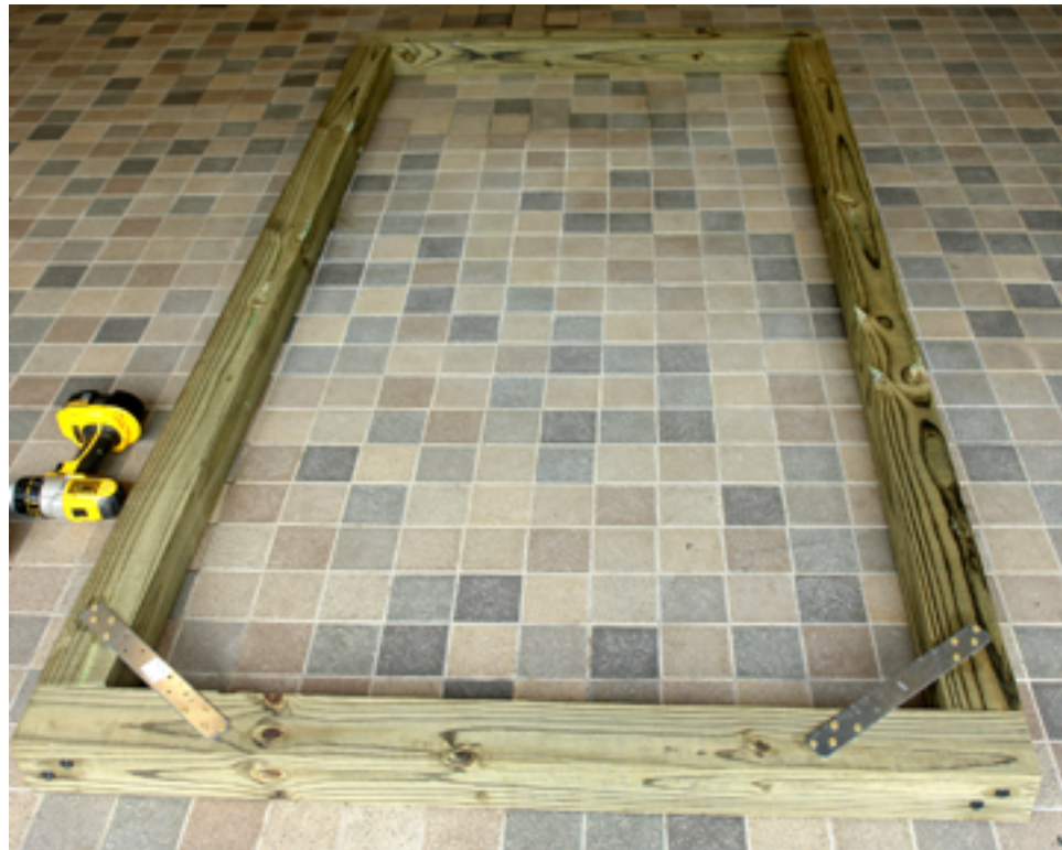
Tunnel Support Fabrication
