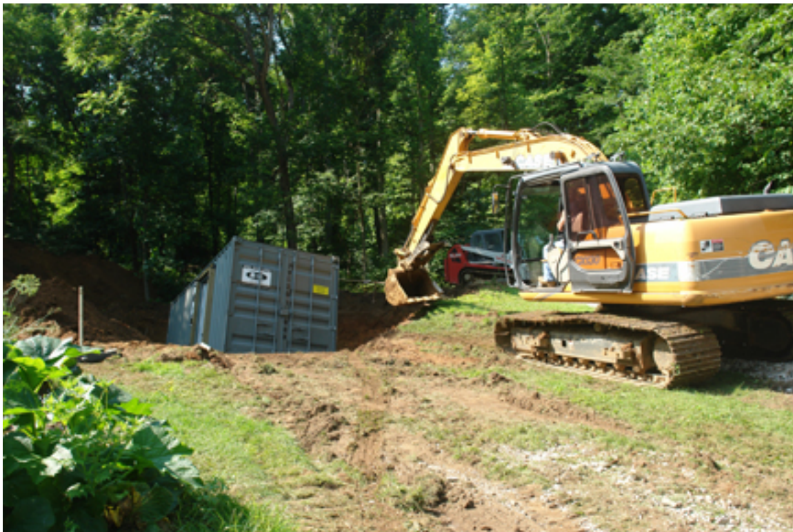
Dragging Shipping Container into Excavation Pit
