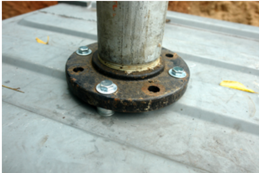
Exterior Flange Attachment
