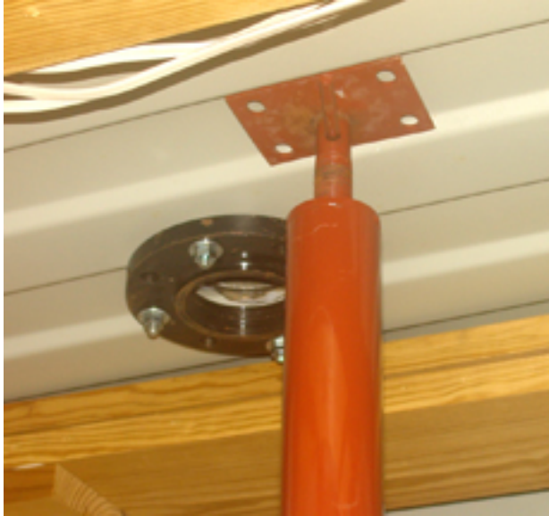
Interior Flange Attachment
