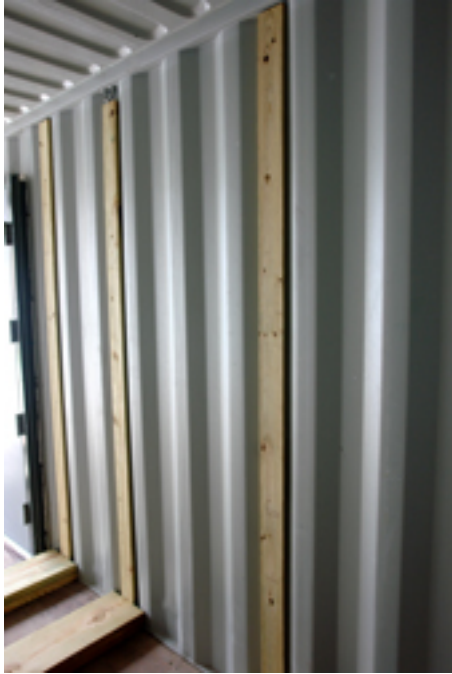
Spacer Board Installation
