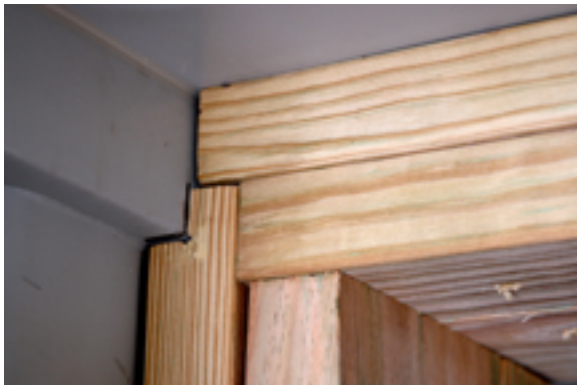
Support Beam Corners
