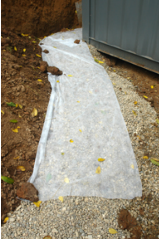
Sediment Shield over Drain Tile
