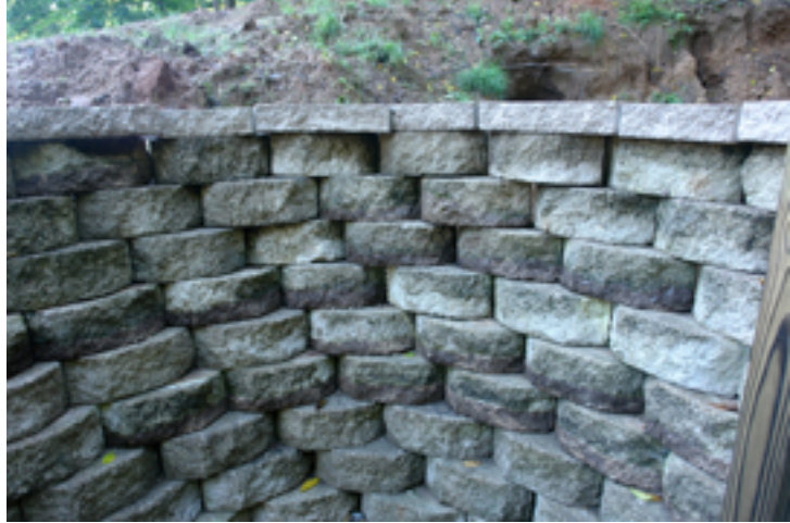
First Layer of Landscaping Blocks
