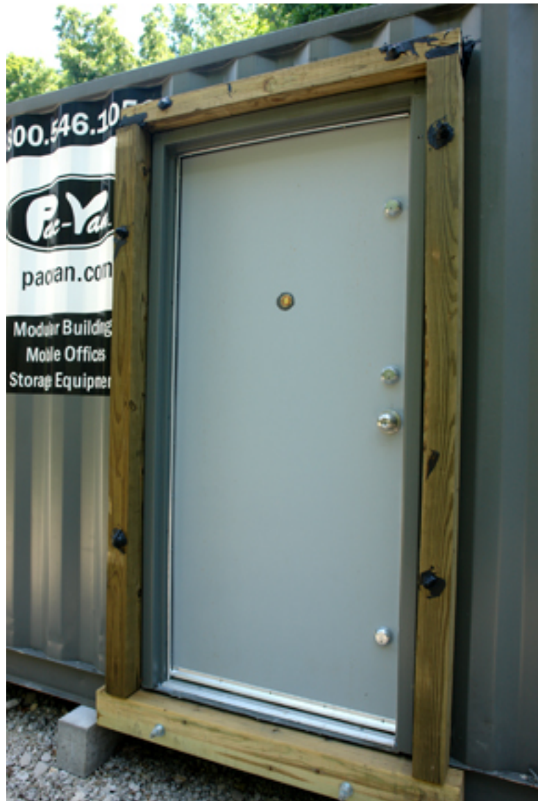
Shipping Container to Tunnel Interface
