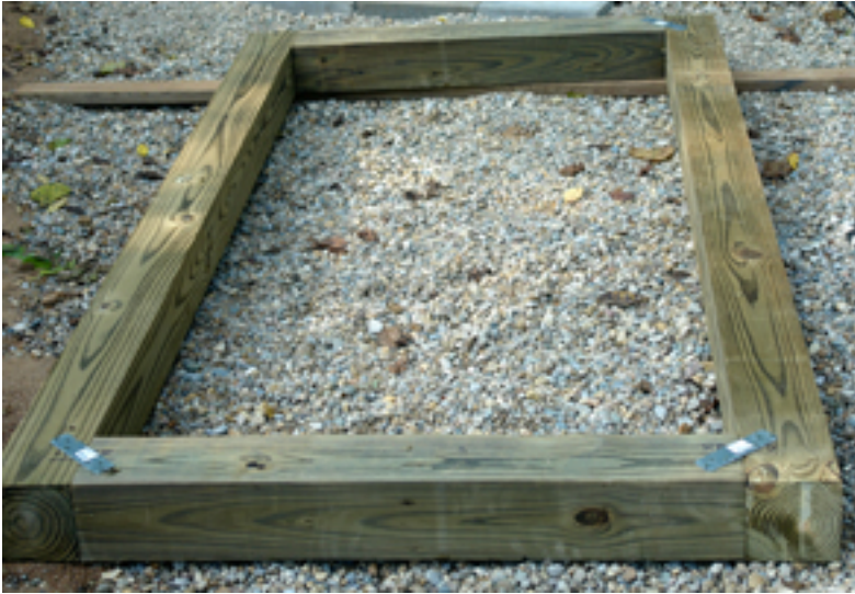
Exterior Doorframe Beam Construction
